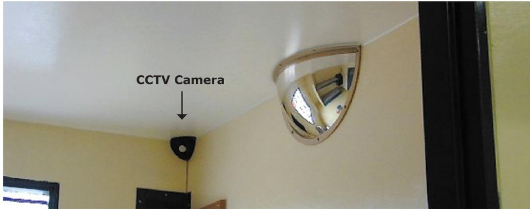
The DuraVision™ Cell Observation Mirror can be used very effectively in conjunction with CCTV. The mirror allows officers to maintain a full visual overview of an area before proceeding. This ensures the officers safety and time is saved as it is not necessary to radio back to the CCTV monitor room for confirmation that it is safe for officers to enter a cell.
